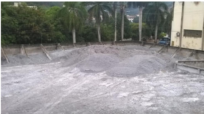
Fig. 1 View of an effluent treatment plant from a pulp paper industry. Source own author
