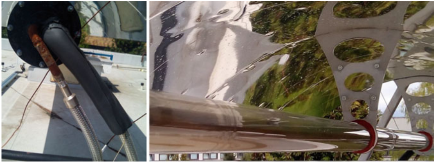
Fig. 3 Detail if inlet/outlet of receiver and reflexive surface
