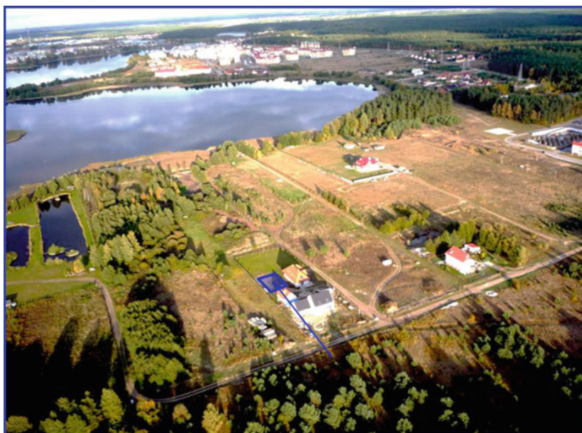
Fig. 1 Location of a ground exchanger nearby Lake (photo by authors)
