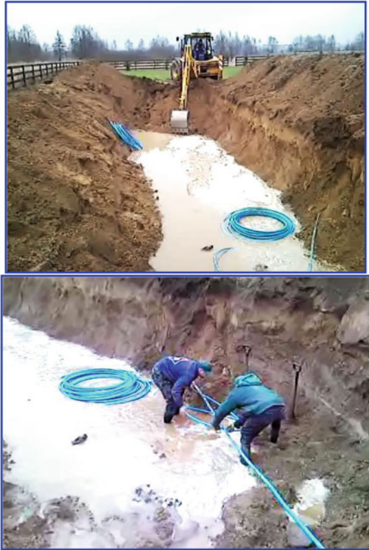
Fig. 2 Laying the ground source heat pump system at a depth of 1.9 m, 10 loops 100 m each, active area of the exchanger is 11 m × 23 m (photo by authors)
