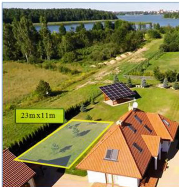
Fig. 3 A view of the area taken by a ground source heat exchanger (photo by authors)
