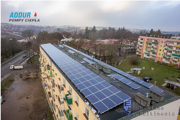
Fig. 1 PV system located on the roof of an apartment building in Szczytno. Source Addur
