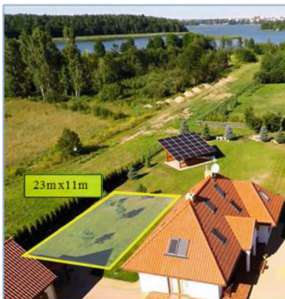
Fig. 3 A view of the area taken by a ground source heat exchanger (photo by authors)
