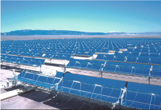
Fig. 4 Solar energy generating station with many arrays of parabolic trough collectors in California [1]
