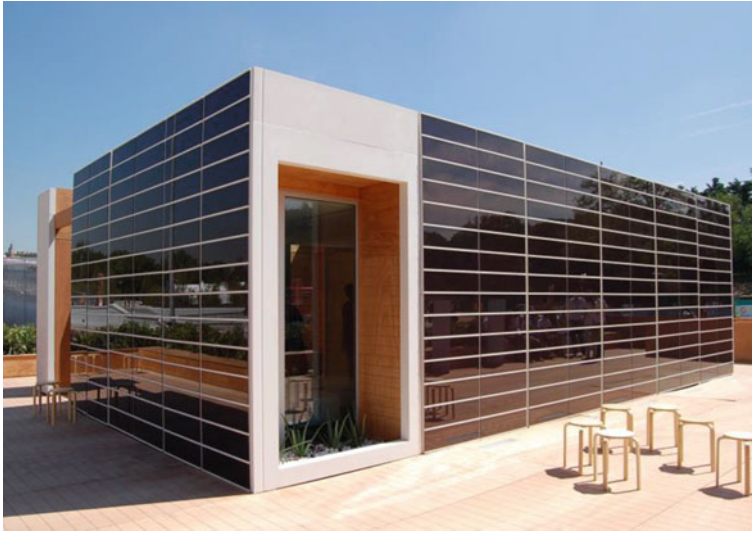
Fig. 4 Elevation created using PV cells. Source ONYX SOLAR BLOG
