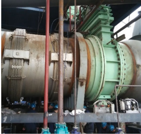
Fig. 13 Optimization of hot blast pipe system compensator
