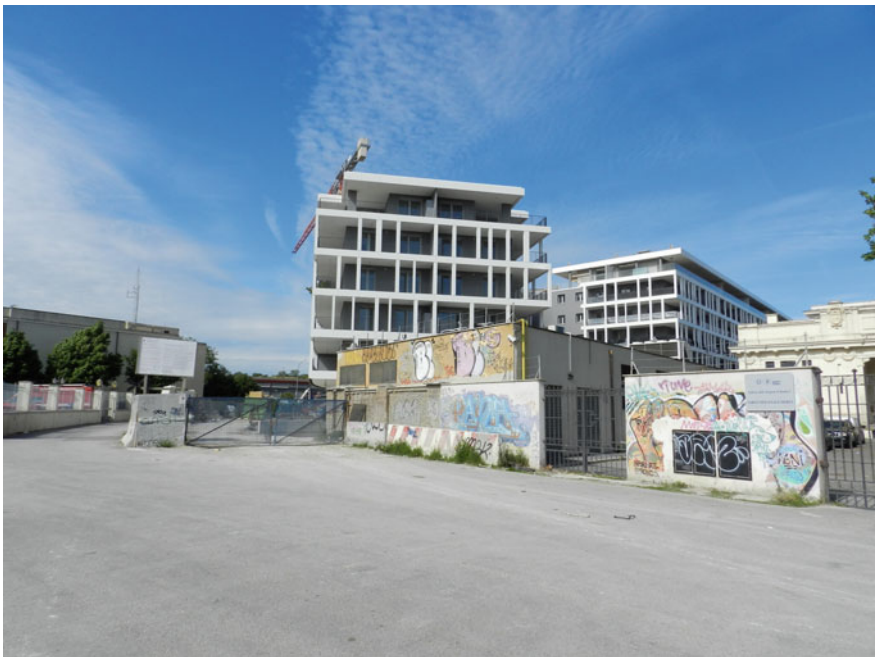
Fig. 3.3 New residential buildings in a multilayered scenario. Published with kind permission of © Nicola Usai 2017. All Rights Reserved
