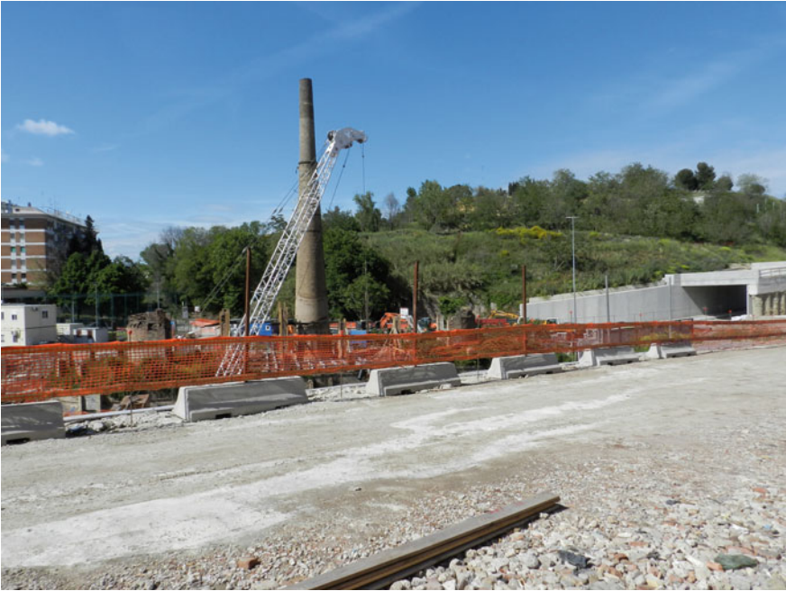
Fig. 2.2 A modern furnace built on top of an antique lime quarry. Published with kind permission of © Nicola Usai 2017. All Rights Reserved
