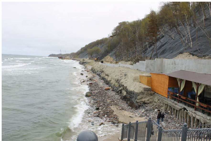
Fig. 3 Construction of the promenade and conducting shore protection works in Svetlogorsk, 2017
