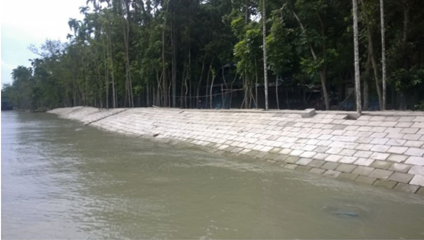
Fig. 19.3 River embankment in Bangladesh. Source Bangladesh Climate Change Trust
