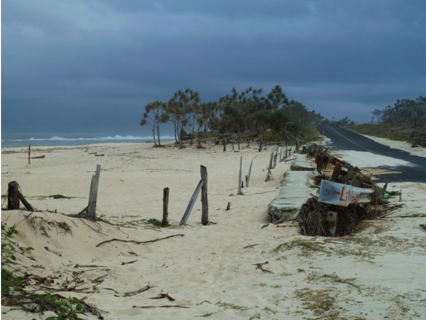
Fig. 15.3 Damage from tropical cyclone Pam in 2015 in north Efate island, Vanuatu. Photo John Handmer
