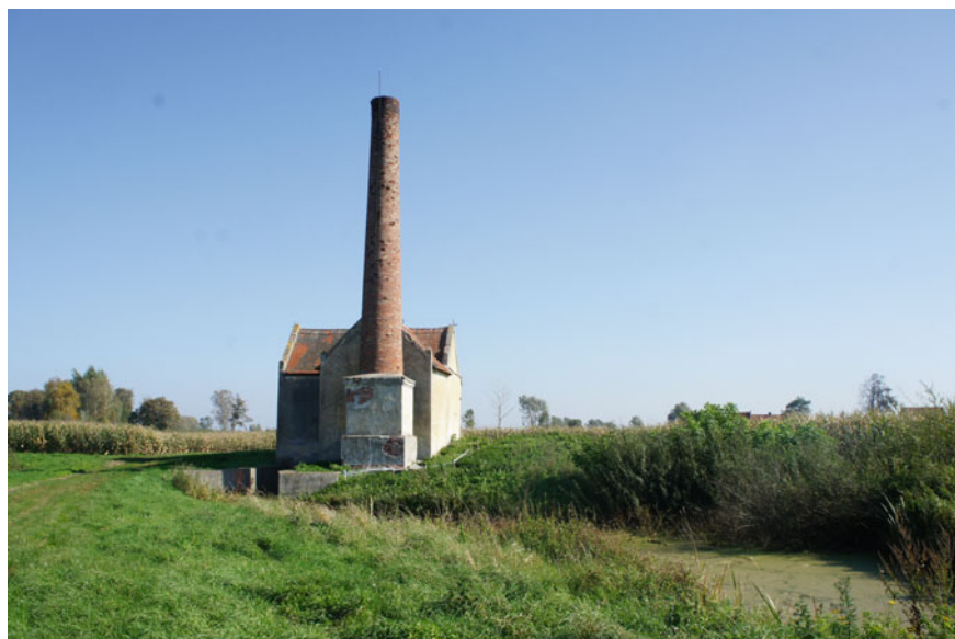
Fig. 6 Historic pumping station in Różany. Photo Klaudia Nowicka
