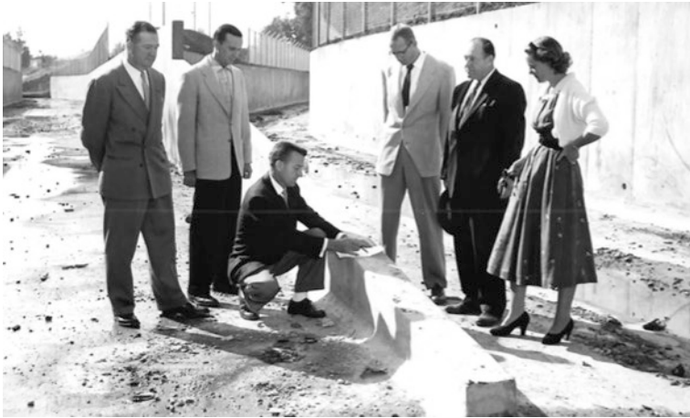
Fig. 5.2 Grayson Creek channel right after completion in 1957 (Courtesy of Contra Costa County Flood Control and Water Conservation District)
