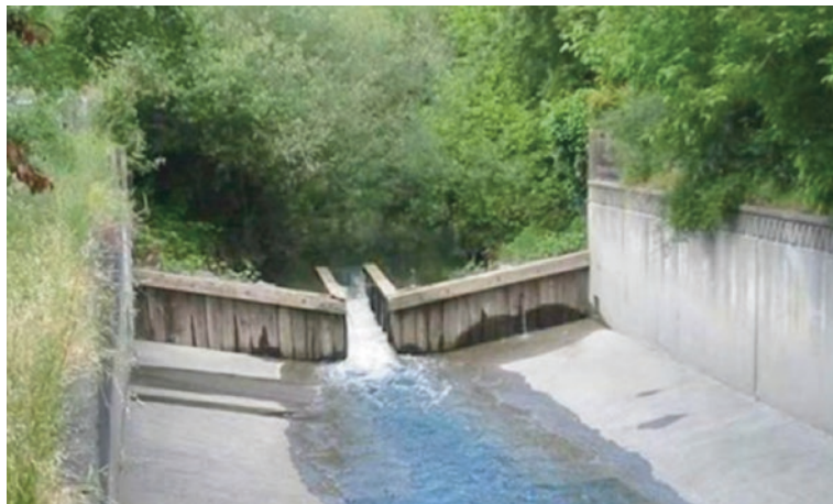
Fig. 5.3 Boundary between Unit 3 and Unit 4 in Ross Creek. Fish ladder separating concrete channel from earthen channel. Unit 4 extends 180 m (600 ft) upstream of this fish ladder (Courtesy of Marin County Flood Control District)
