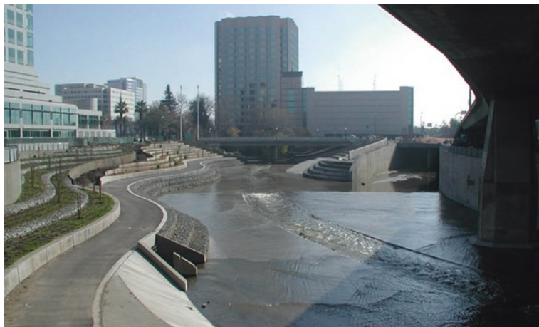
Fig. 5.5 Guadalupe River flood control project looking upstream at outlet of Woz Way Bypass, downtown San José, California (Courtesy of Marin County Flood Control District, 2006)
