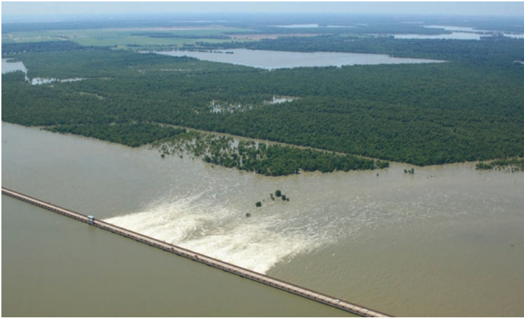
Fig. 2.3 Morganza Floodway in operation during the 2011 Mississippi flood (Source: US Army Corps of Engineers)
