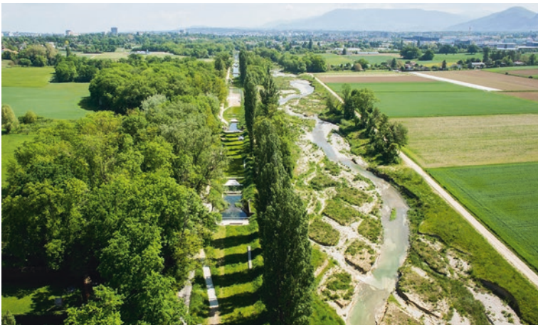
Fig. 6.3 View eastward of the Aire River in May 2016, showing the repurposed nineteenth-century canal on the left and the new river corridor on the right (photo by Fabio Chironi ©, used by permission)
