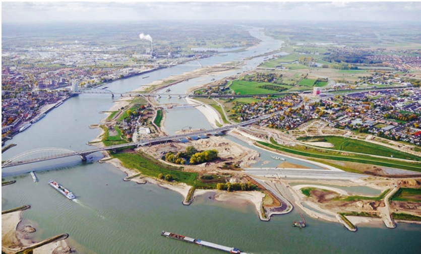
Fig. 4.3 River widening and waterfront redevelopment at Nijmegen/Lent, the Netherlands. View from 2015 showing project nearing completion, with broader river channel, and diversion channel, new waterfront, road, bridge and rail infrastructure (Courtesy of Johan Roerink and H+N+S Landscape Architects)
