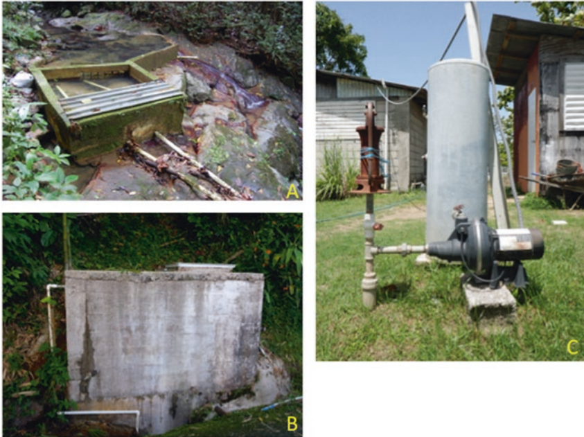
Fig. 22.2 Examples of surface (A, B) and underground (C) rural water systems. In (A), a typical stream water-collection point, the community has constructed a small ditch and connected a PVC pipe. (B) is an example of a spring water collection system. The community constructs a box around a spring and the water is transferred to a collection tank. (C) is an example of a groundwater pump. Most non-PRASA systems transfer the water from the collection point to a tank where the water is chlorinated and distributed. However, some households within the community and some entire communities consume the water directly from the source
