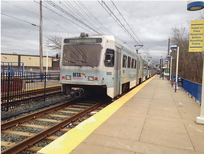
Fig. 43.4 MTA Light Rail Station in Timonium, Maryland
