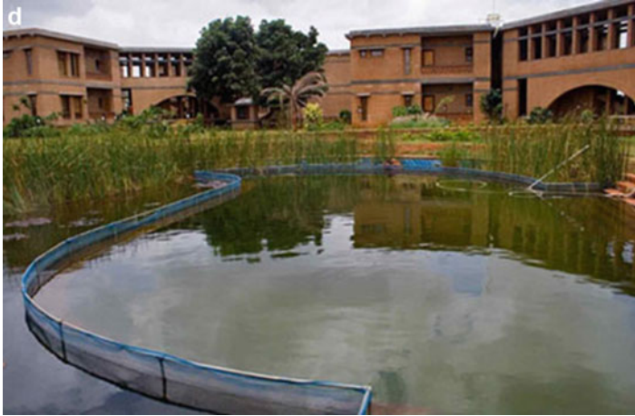
Fig. 5 (a–d) Phases in construction of the bio-pool
