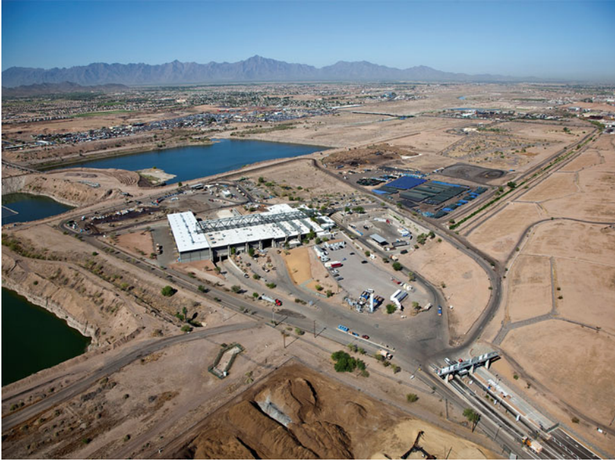
Fig. 2 The Phoenix 27th Avenue Waste Transfer Station, home to the Resource Innovation Campus and RISN (Photo courtesy of City of Phoenix Public Works Department)
