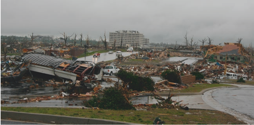
Fig. 3.1 St. Johns Hospital following 2011 tornado. Photo courtesy of the City of Joplin
