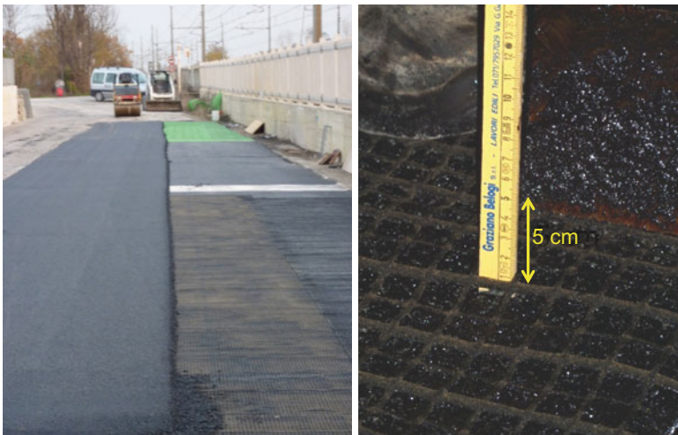
Fig. 4.19 Laying of the AC12 upper layer
