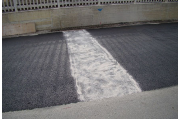
Fig. 4.18 Polymer modified tack coat and artificial debonding with fine sand
