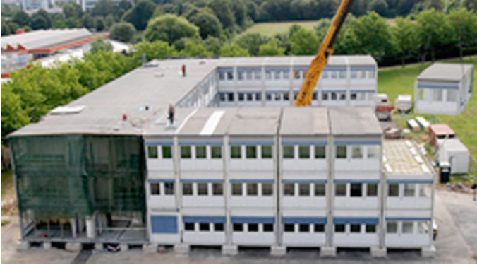
Fig. 39.1 A part of Bielefeld University is built from the container modules Courtesy by Norma Langohr
