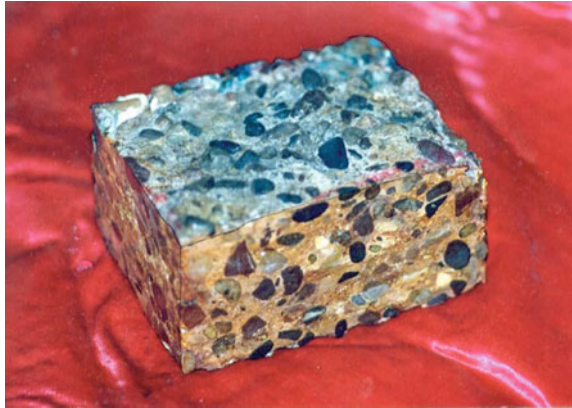
Fig. 6.2 Concrete from the water storage tank of ancient city of Camiros (Efstathiadis 2004)
