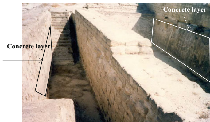
Fig. 6.1 Water storage tank in the ancient city of Kamiros, Rhodes, Greece. Concrete layers were used as water sealers. The water tank was put out of order during the 3rd century BC due to the construction of a Doric Portico with foundations of 1.60 m × 200 m (Efstathiadis 2004)
