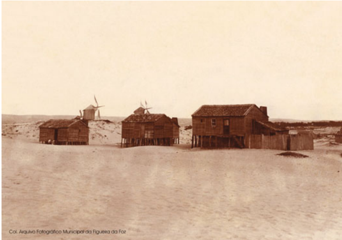
Fig. 1 Palheiros from Costa de Lavos (Figueira da Foz). Photo from the Photographic Archive of the Municipality of Figueira da Foz
