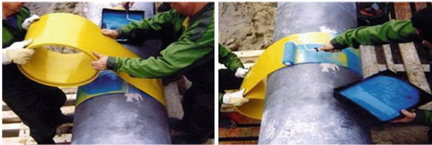
Fig. 6 Clock Spring® sleeve being applied to a damaged, steel pipe
