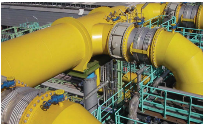
Fig. 1 Refinery expansion joint
