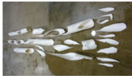
Photo 5. PVC pipe failure
