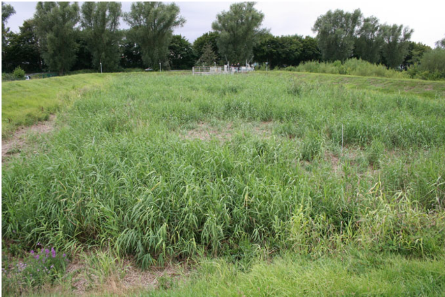
Fig. 2.10 Bioretention filter (2200 m 2 ) for the treatment of pre-settled CSOs in Germany (Photo K. Tondera)
