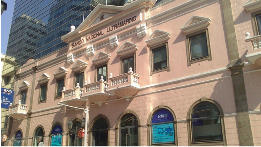
Fig. 2 The façade of Banco Nacional Ultramarino with new glass high-rise add-on tower
