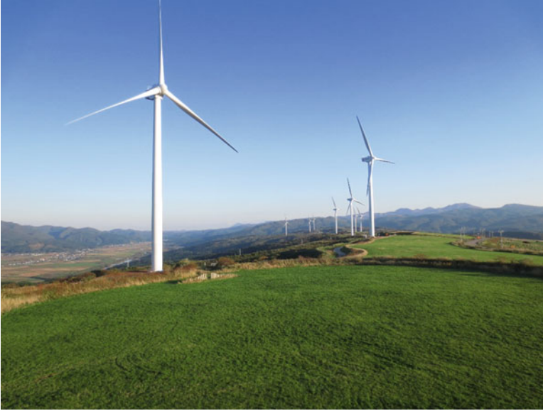
Fig. 39.1 Kaminokuni wind farm, in Hokkaido, 28 MW, MHI 2.4 MW \times 12 units, ©J Power
