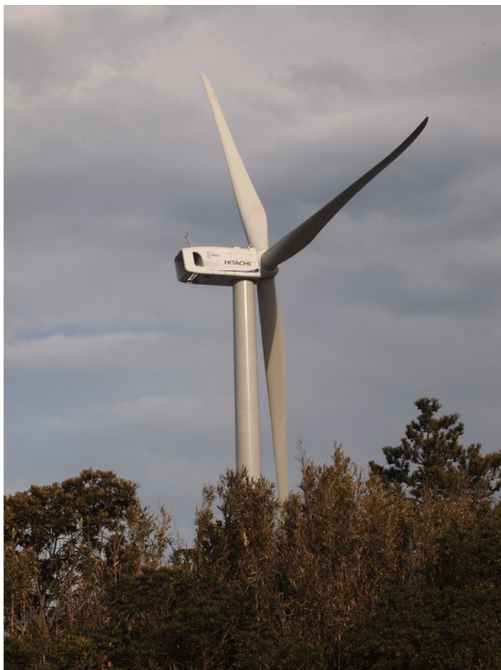
Fig. 39.2 Hitachi's HTW5.0-126 5 MW turbine at Kashima port side ©Hitachi
