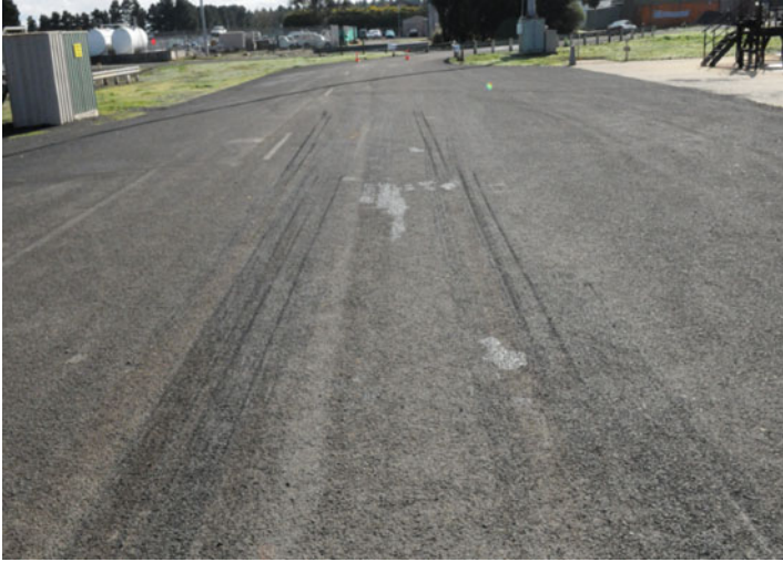
Fig. 8.16 CFA Training Facility, Fiskville, looking north on testing field
