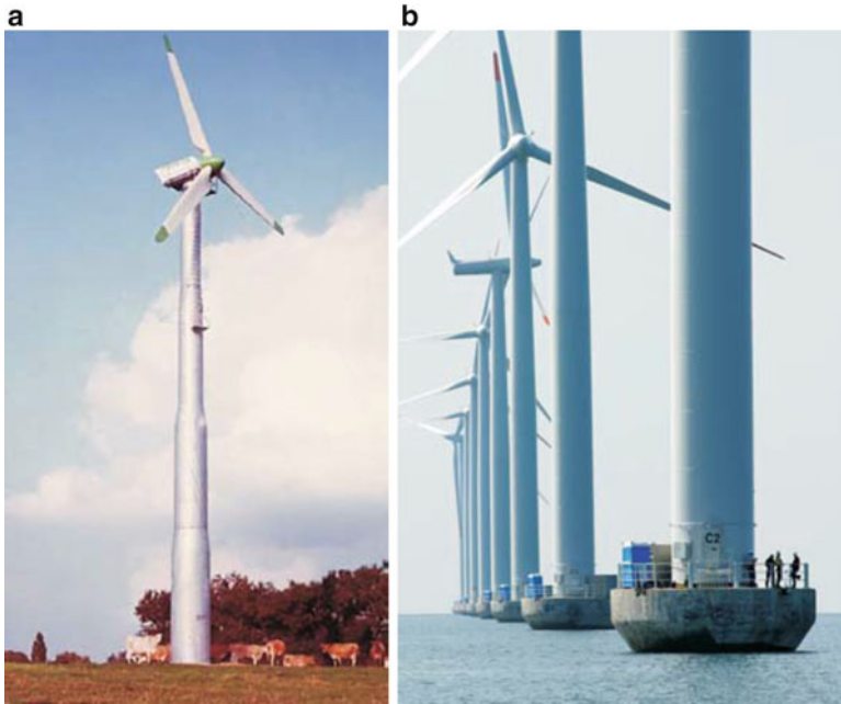
Fig. 1.3 (a) Single wind turbine of 30 KW used in the 1980s (Larsen 2005). (b) Arrays of HAWT of 2.3 MW each at the shores (Larsen 2005)
