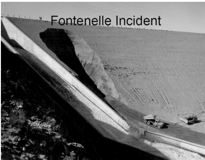
Fig. 5.11 Piping in dam face (Snorteland 2013)
