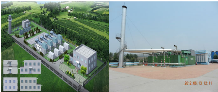
Fig. 22 Picture of the landfill gas power plant of XiaoJianXi. Note: The images were provided by the “DongJiang Environmental Renewable Energy Co., Ltd of Qingdao”
