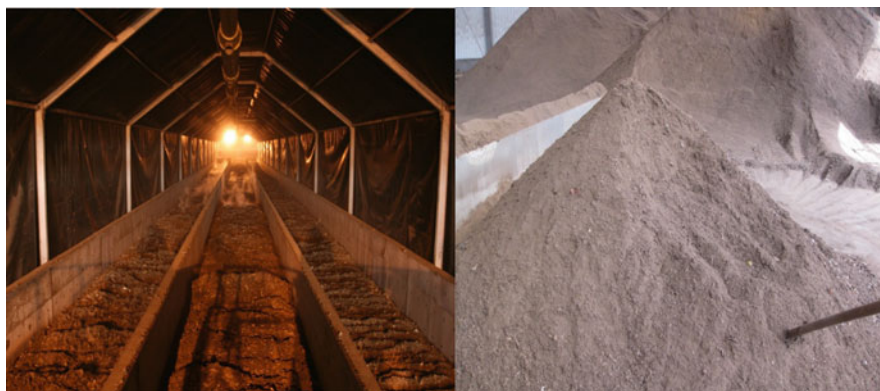
Fig. 20 Compost fermentation room and compost product. Note: The images were provided by the “MSW biochemical treatment plant of XiaoJianXi”
