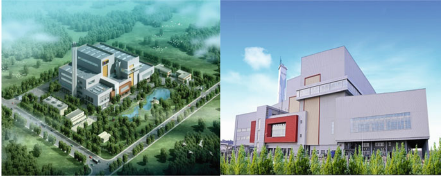
Fig. 17 MSW incineration power plant of XiaoJianXi. Note: The images were provided by the “Environment Renewable Energy Co., Ltd of Qingdao”
