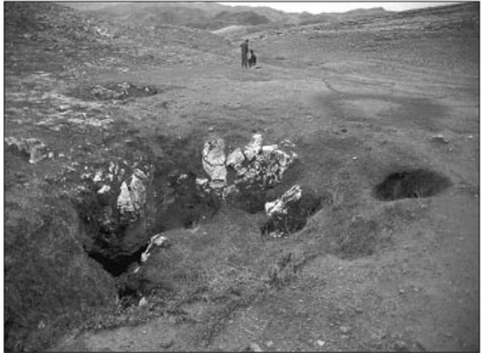
Fig. 4.3 Sinkhole opening in residual soils near the Karkheh River (after Cucchi and Zini 2003)
