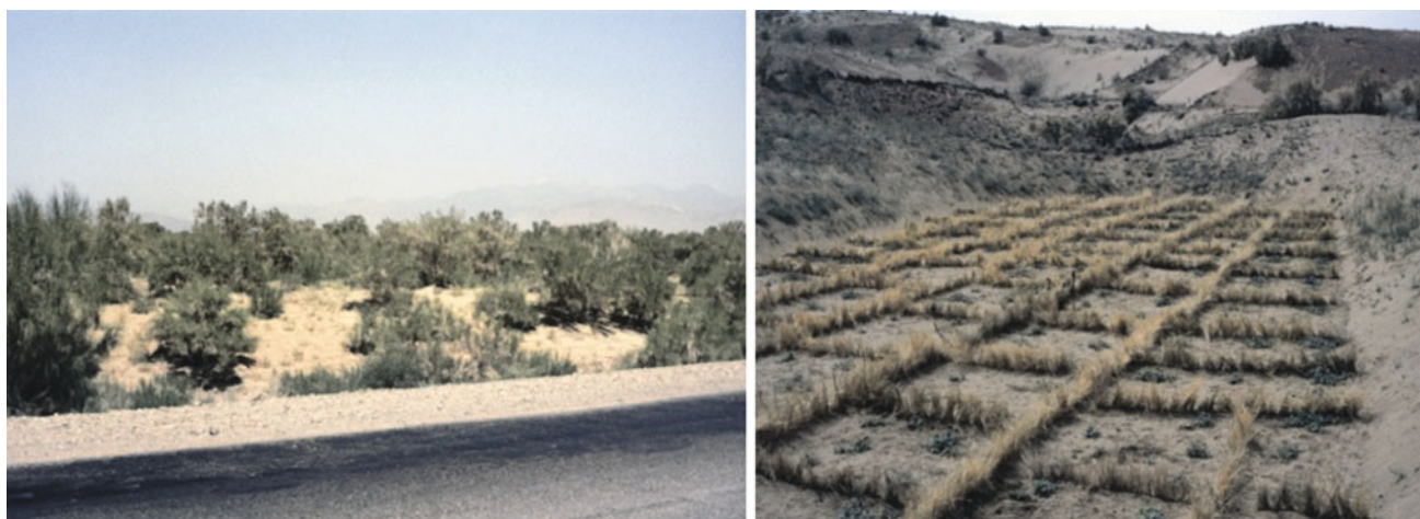
Fig. 14.1 Sand dune stabilization in Kashan, Yazd, and Kerman: good projects, but not properly coordinated or continuously supervised (Farshad 1997)
