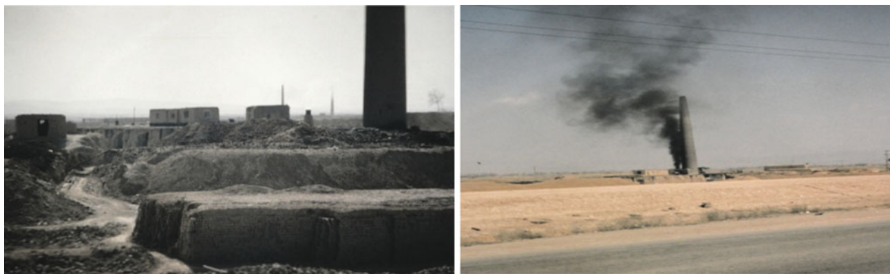
Fig. 14.6 Prime agricultural soils are used in brick-making factories, an example from Hamedan Province (Farshad 1997)
