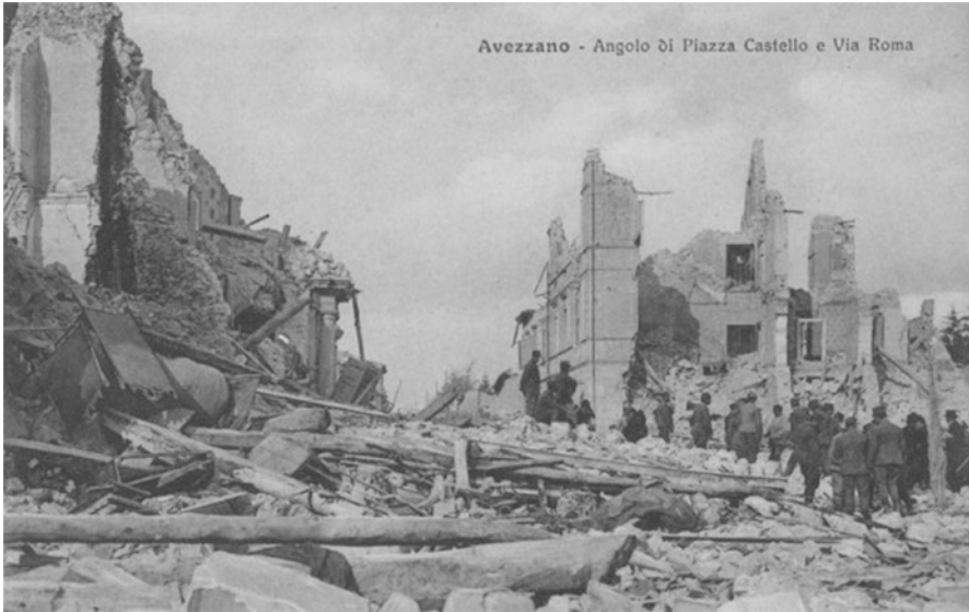
Fig. 18 Postcard of Avezzano after the earthquake
