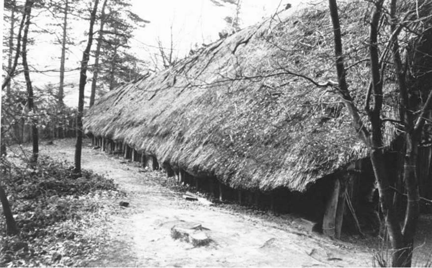
Fig. 4.11 Reconstruction of a Neolithic Linear Pottery longhouse of the Rössen Culture in the Oerlinghausen open-air museum near Bielefeld. These thatched oak constructions could reach a length of 40 m and accommodated clans and their domestic animals. These buildings were not infinitely long-lived and devoured a tremendous amount of wood in the heretofore primeval landscape's first cleared islands
