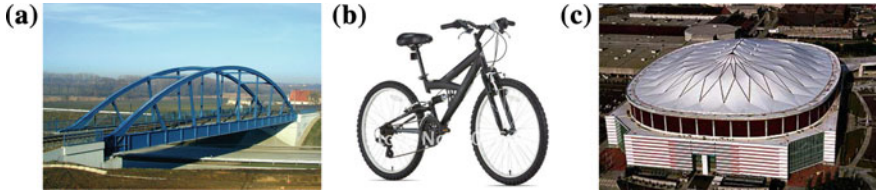
Fig. 1 Structures are typically composed by interconnected rigid bodies and they can have different types of mobility. a A fixed bridge is an example of rigid structure. b The shock absorbers of a bike are passive mobile structures. c Retractable roofs are active structures
