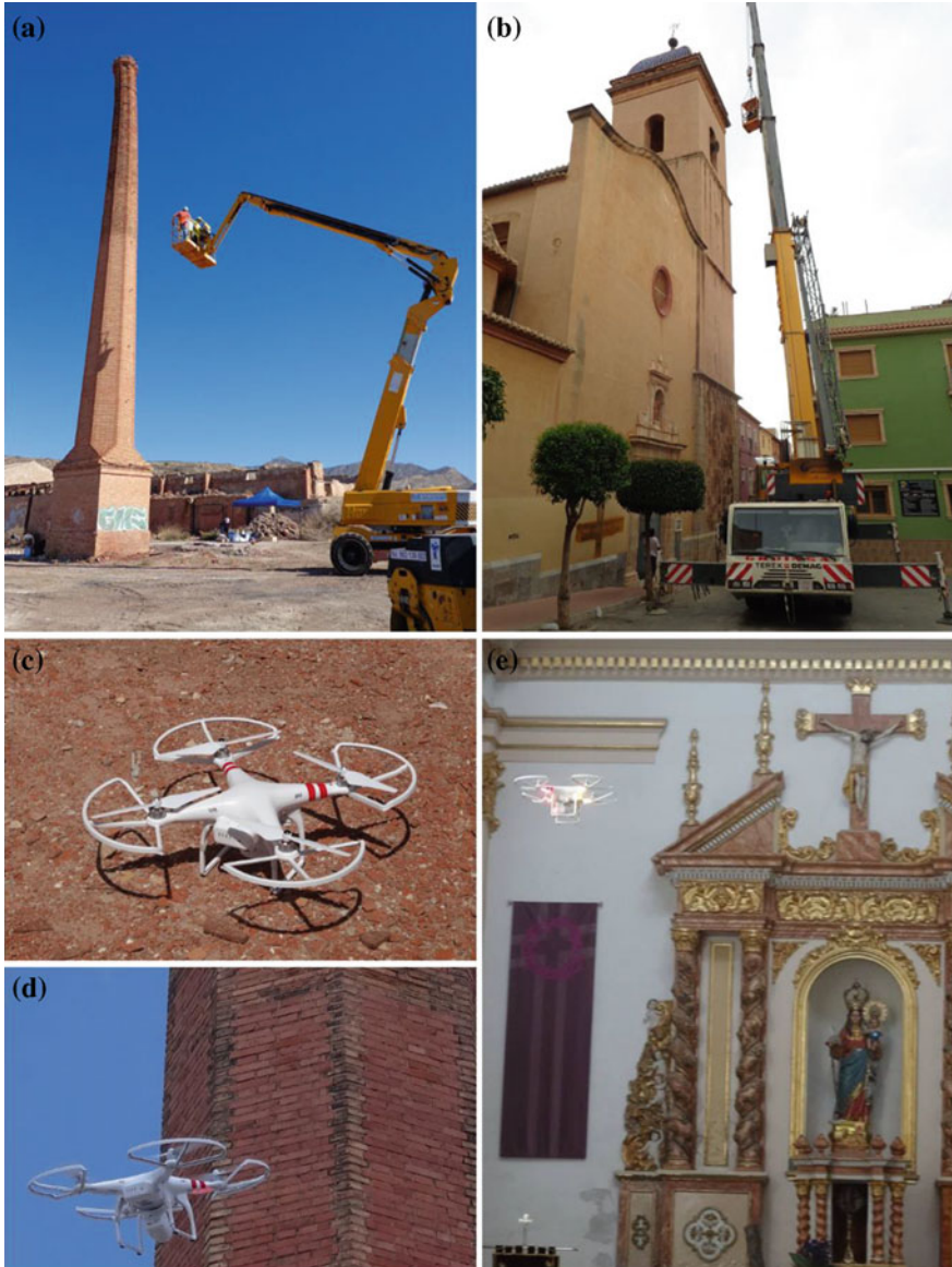
Fig. 2 Human visual inspection: a masonry chimney and b bell tower, both protected structures in Agost (Alicante). c UAV for automated inspection used in d masonry chimney and e interior inspection of Saint Peter's Church, both in Agost
