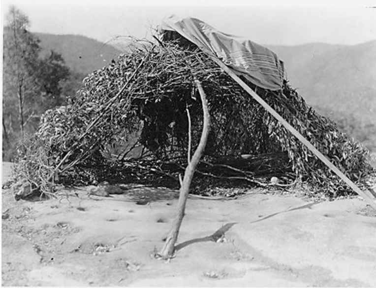
Fig. 4.6 Chaparral brush was used extensively for different types of structures and fencing. One example is the building of shade structures such as this brush structure designed to shield North Fork Mono women from the sun as they pounded acorn and other foods in mortar holes in a granite outcrop, North Fork, Madera County, California. Museum Number 15-6221, courtesy of the Phoebe A. Hearst Museum of Anthropology, UC Berkeley
