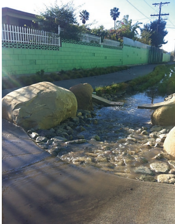
Fig. 8.4 An example of “green infrastructure” in the City of Sun Valley, California. Surface runoff from an adjacent residential street is directed into this constructed bioswale to improve water quality by naturally removing contaminants in the water as it percolates into the soil. Photo by Eileen Alduenda
