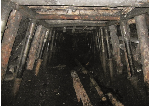
Fig. 5. Face No.2 with hydraulic props (photo courtesy of Long Quoc Nguyen)
