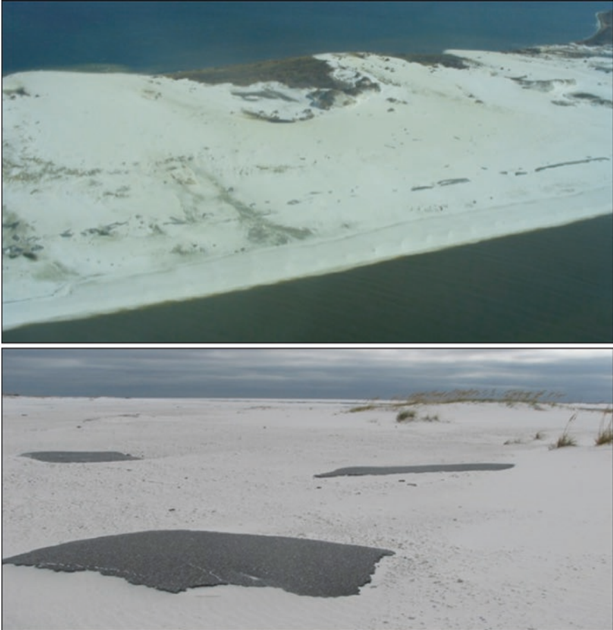
Fig. 11 Damage to road on Santa Rosa Island following Hurricane Ivan. Damage to the road was extensive in the narrow sections of the island (between headlands) leading to a lag of shell, gravel, and asphalt that further limited dune recovery (Houser 2009)
