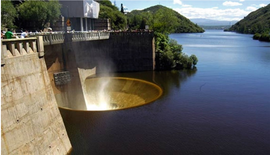
Fig. 8 View of the morning glory spillway of the San Roque Dam
