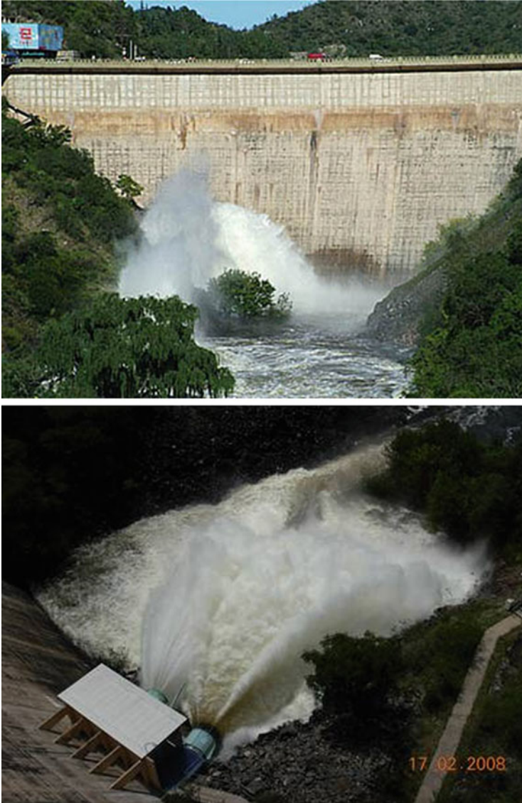
Fig. 7 View of the discharge and discharge valves of the irrigation intake (2008)
