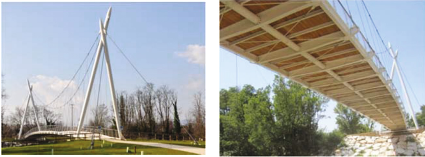
Fig. 1. Seriate footbridge: (a) overall view; (b) footbridge deck, detail of longitudinal and transverse beam.
