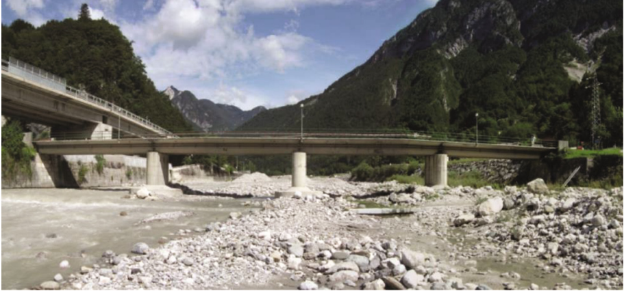
Fig. 5. Dogna bridge, Italy.
