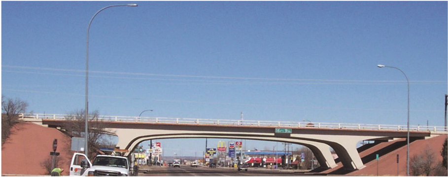
Fig. 1. Bridge 7937 in Tucumcari NM.
