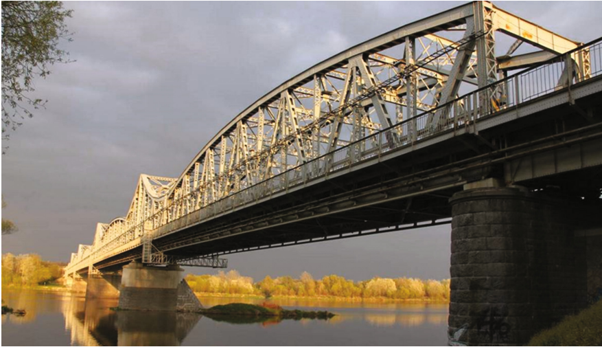
Fig. 1. The Ignacy Mościcki Bridge over the Vistula River in Puławy
