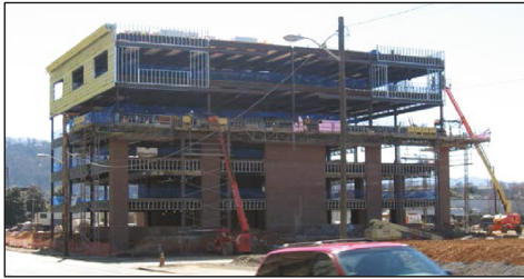
(a) As-Tested Building Condition
