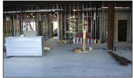
(b) As-Tested Floor Condition
