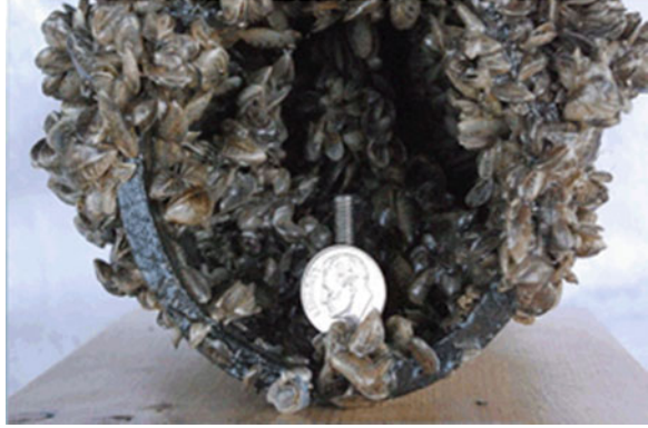
Fig. 3 Zebra mussels attached to a pipe (Photo from Mussel Prevention Program, San Luis Obispo County, California)
