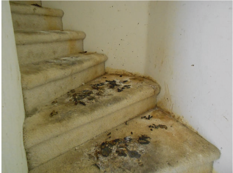
Fig. 3.26 Entryway into home of the second floor condominium
