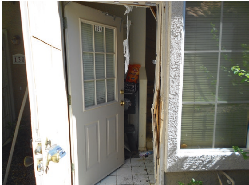
Fig. 3.25 Forced entry into the house of a hoarder by police
