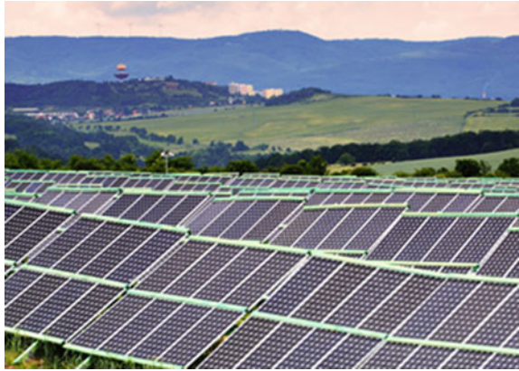
Fig. 2.4 A photo of a typical solar-power plant ( http://www.publicdomainpictures.net/view-image.php?image=30618&picture=solar-power-plant )
