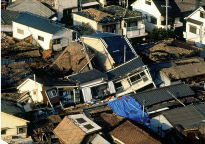
Fig. 2.7 Collapsed houses in Kobe caused by the 2002 earthquake ( http://images.nationalgeographic.com/wpf/media-live/photos/000/002/cache/kobe-house-collapse_262_600x450.jpg )
