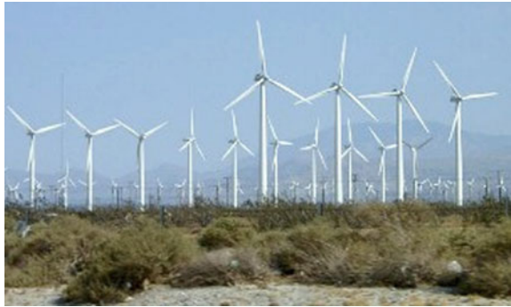
Fig. 2.5 An example of a wind-power-generator “farm” ( http://www.worsleyschool.net/science/files/windpower/page.html )
