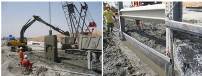
Fig. 1 Excavation of a trench
