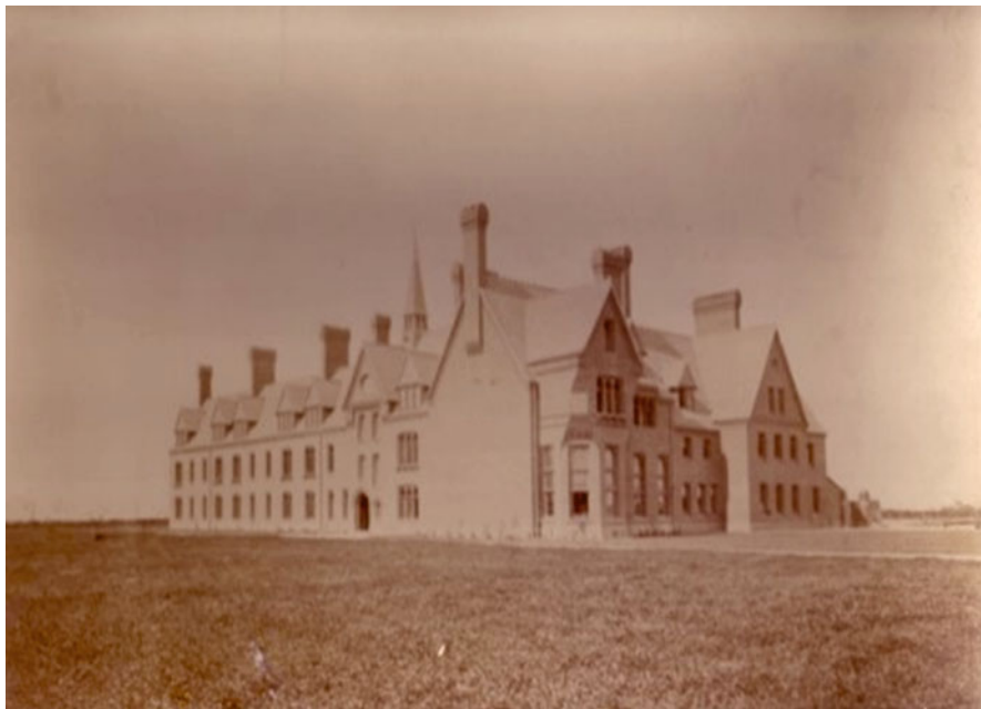
Fig. 1.1 Photograph of the first building, now part of the Old Wing, circa 1872. Courtesy of the Mistress and Fellows, Girton College, Cambridge.
