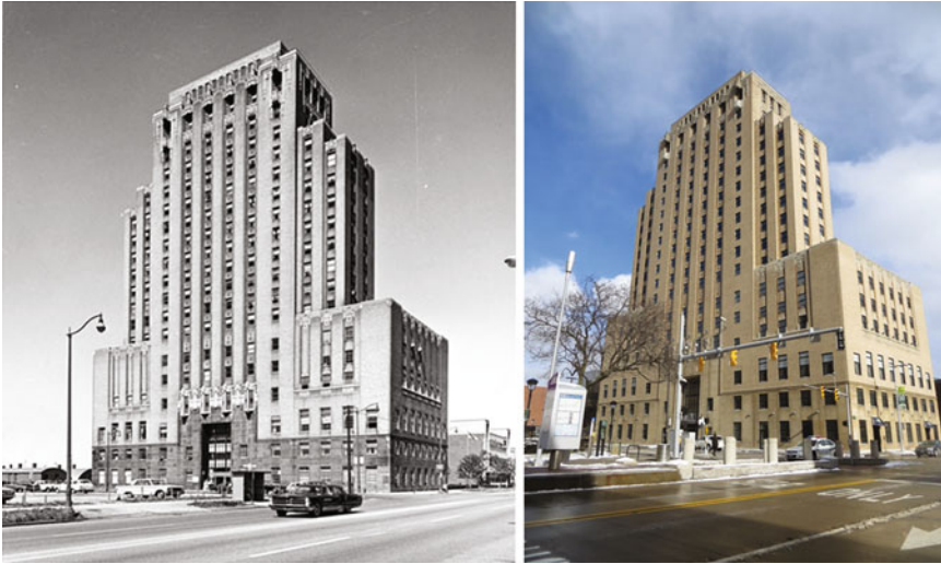
Fig. 2.1 Fenn Tower before restoration c. 1965 ( left ) and after the 2006 restoration ( right ). Source: https://www.google.com/search?q=Fenn+Tower&rlz=1C1GPEA_enUS315US382&espv=2&biw=1024&bih=677&tbm=isch&tbo=u&source=univ&sa=X&ved=0ahUKEwiI1vqVjOLNAhVCWSYKHUbuBksQ7AkIQA&dpr=1
