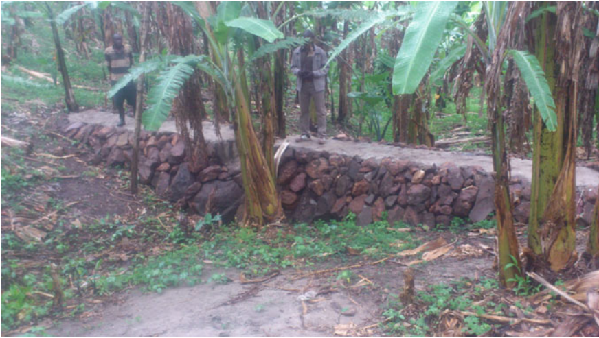
Fig. 4 A check dam in a banana garden. Photo James W. Kisekka
